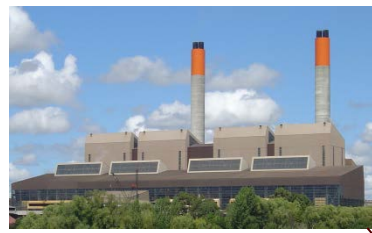
Coal-fired generating plant
