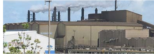
Glenbrook steel mill co-gen
