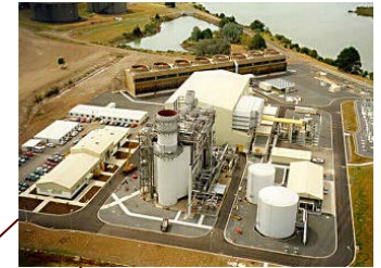
Gas-fired generating plant
