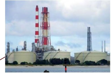
Marsden Point oil refinery
